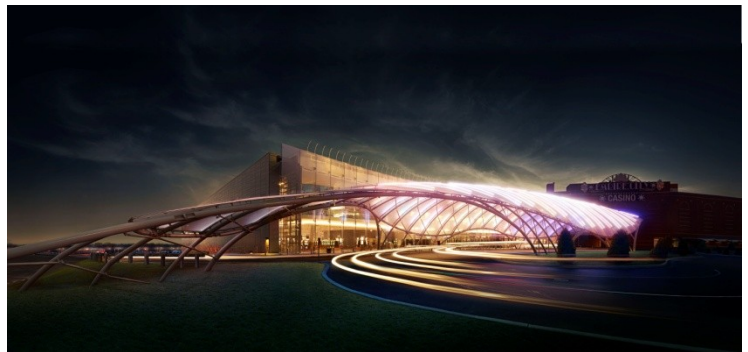
Exterior – Empire City Casino
